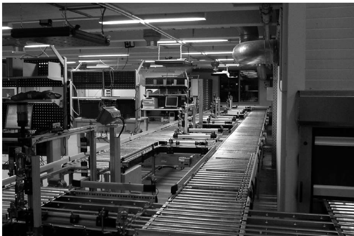
... conveyor technology at Airport Frankfurt.
